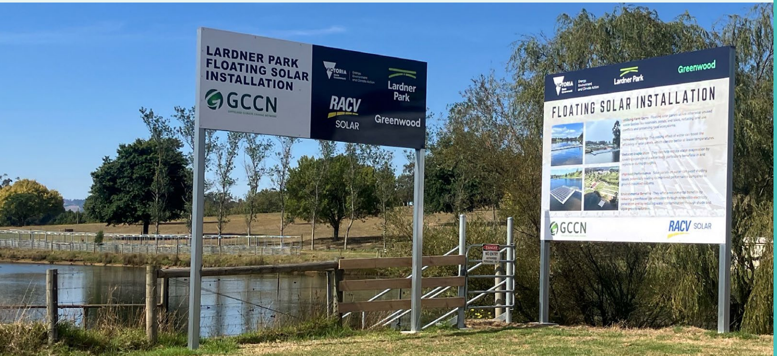
Photo: Floating solar photovoltaic system at Lardner Park.
